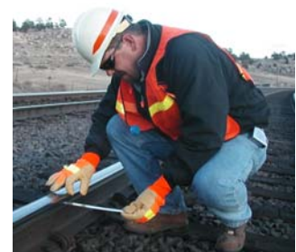
The FRA National Inspection Plan directs safety inspectors to potential “hot spots.”
